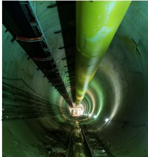
23ft ID Northeast Boundary Tunnel
