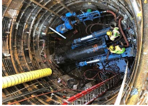
Microtunneling Launching Shaft
