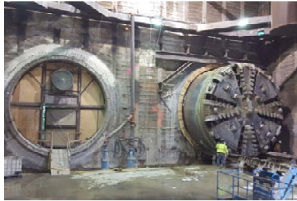
TBM Breakthrough at Crenshaw/Vernon Underground Station
